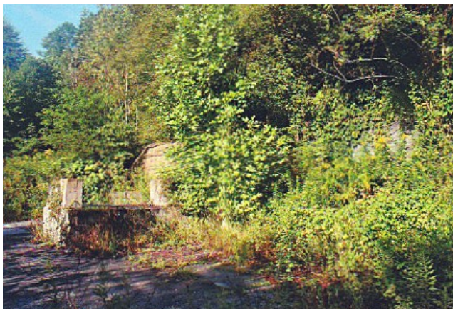
Cranberry Forge Foundations
